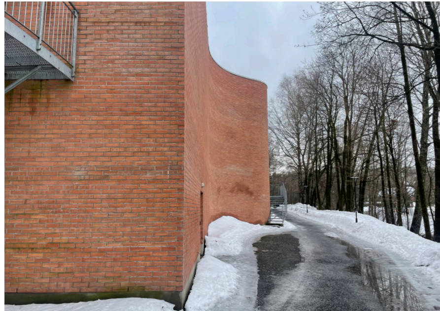
Existing structures - Sandvika High School
