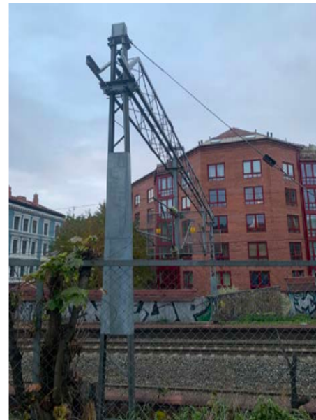
Supporting the supports
