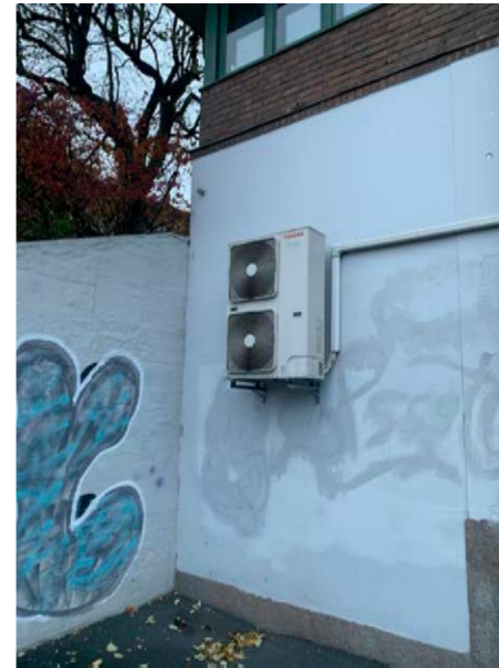
Outlet from the building's organs
