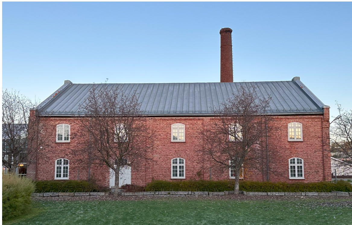
East facade, Saw building
