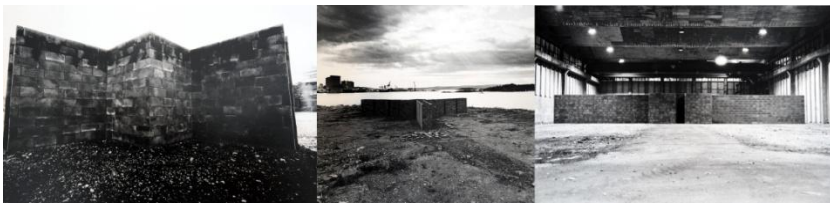
Figure 1-1 Three different large scale structures built by Leca concrete blocks, 1990.
